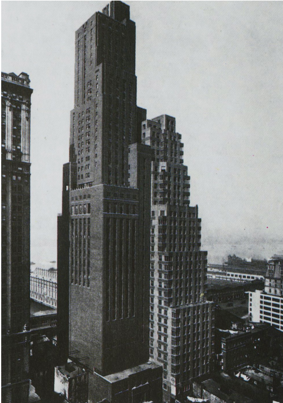
Downtown Athletic Club, 1931 (Starrett & Van Vleck, architect; Duncan Hunter, associate architect). Successful lobotomy made this apotheosis of the Skyscraper as instrument of revolutionary metropolitan culture almost indistinguishable from surrounding Towers.
