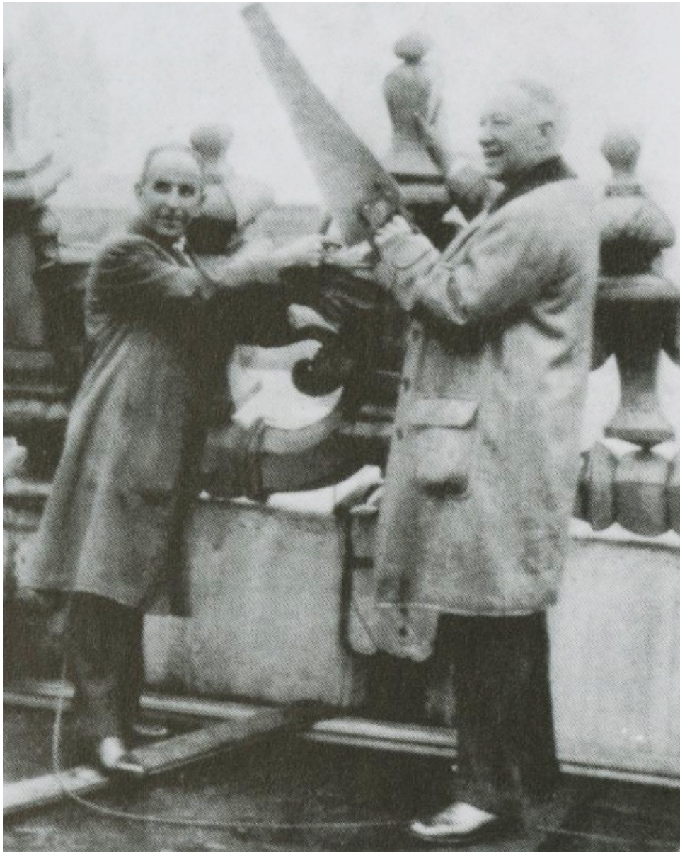
"Messrs. Raskob and Smith begin to demolish the Waldorf..."
