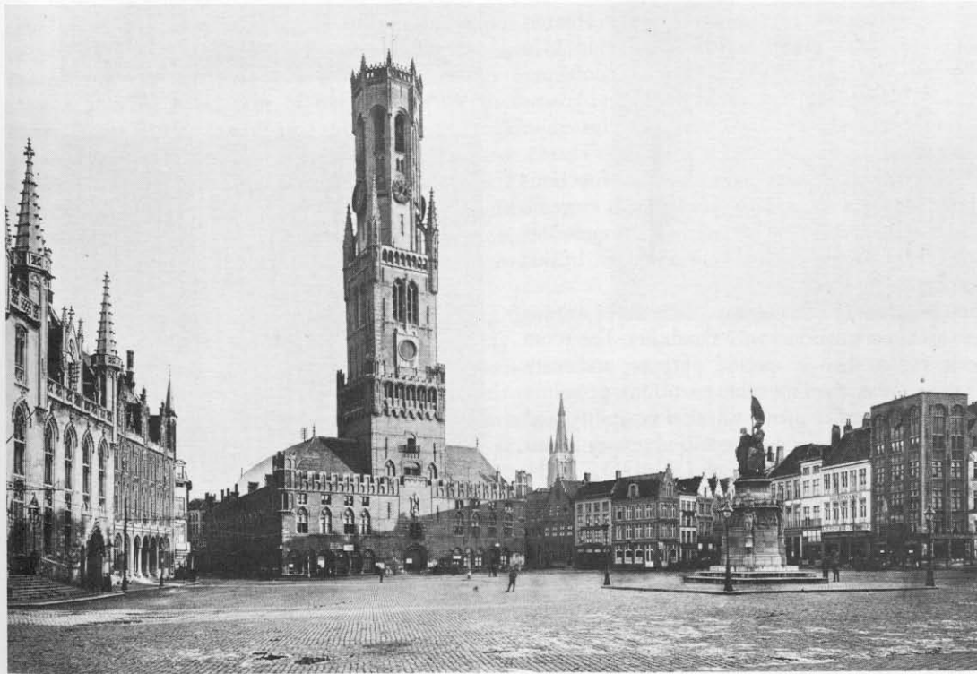
40. Cloth Hall and Belfry, Bruges
